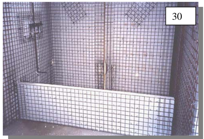
This bathtub that will be later covered in concrete and finally with ceramic tile has been perfectly assembled with 3-D panel.
